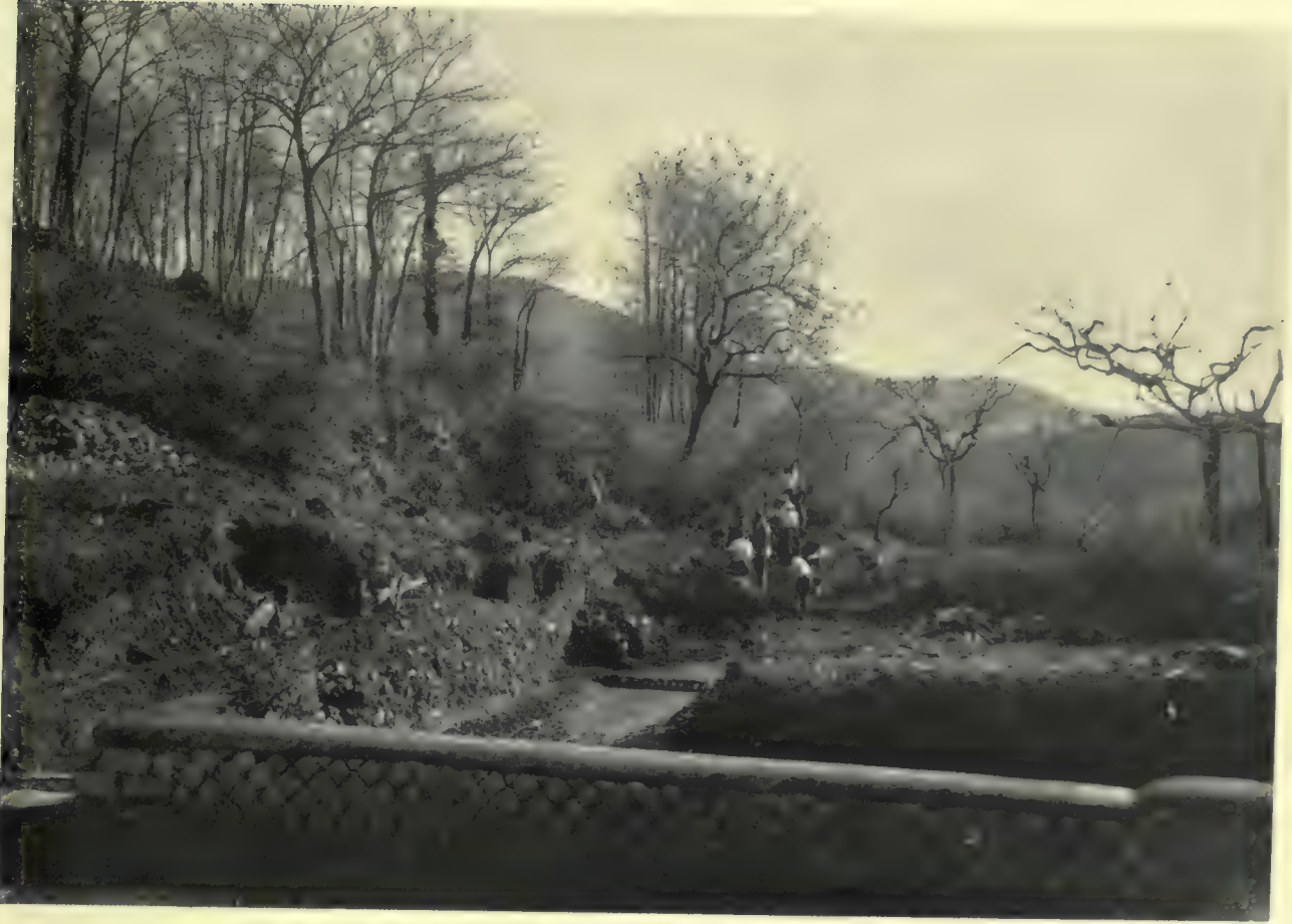
1. New Excavation of East Porticus, from Northwest.
